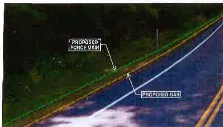
Figure 2 - Schematic gas and force main layout
